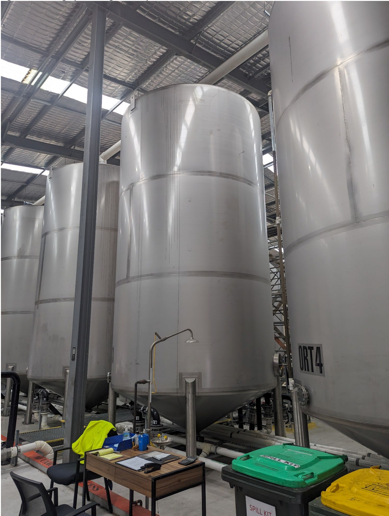
Figure D6. Photograph of the grease trap and food waste tank farm.
