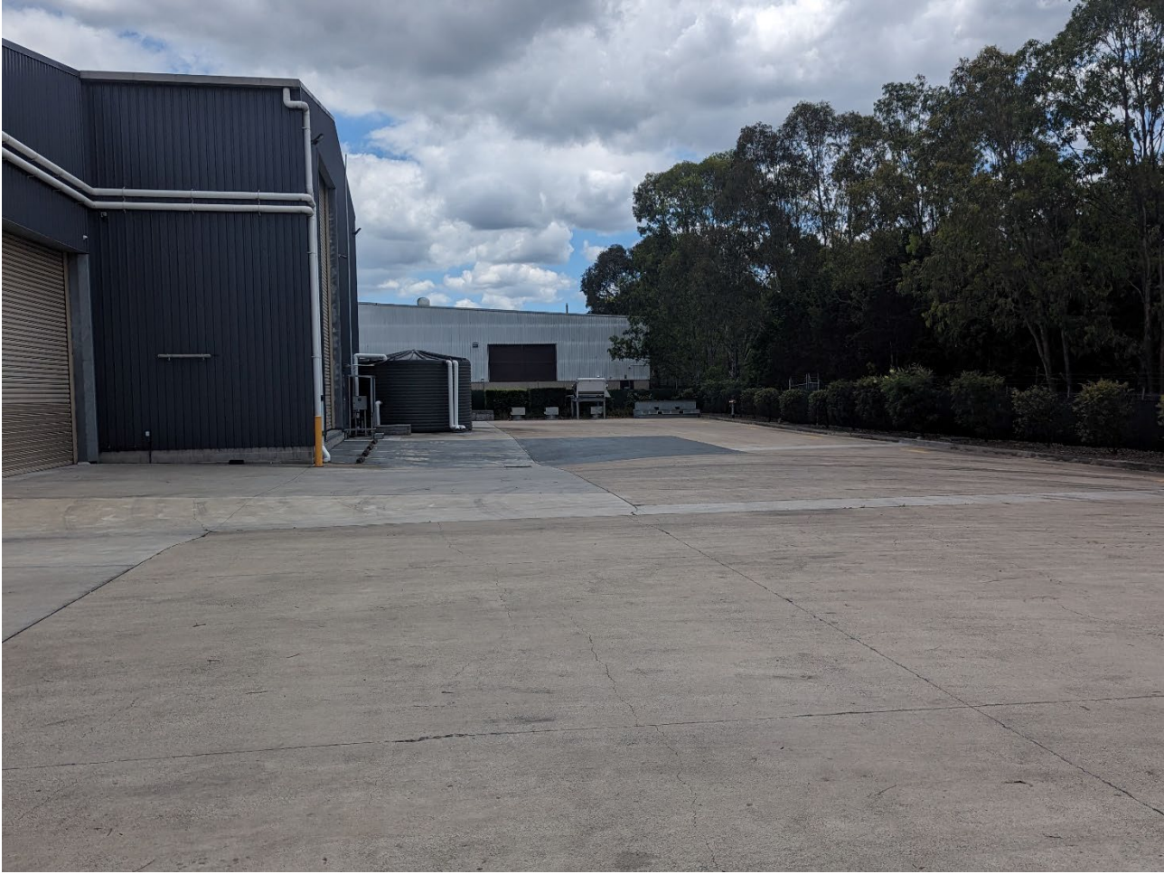
Figure D9. Photograph of the rear of the Site.
