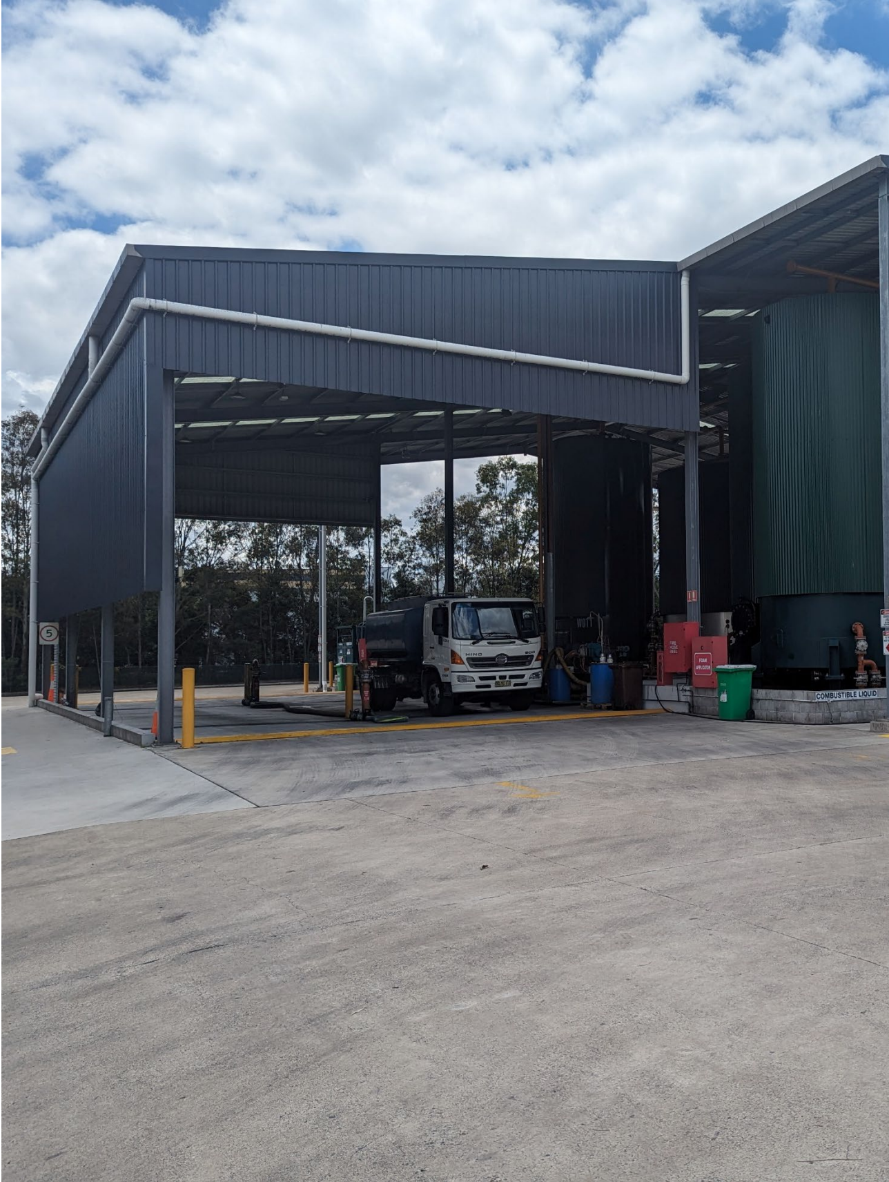
Figure D7. Photograph of the used oil loading and unloading bays.
