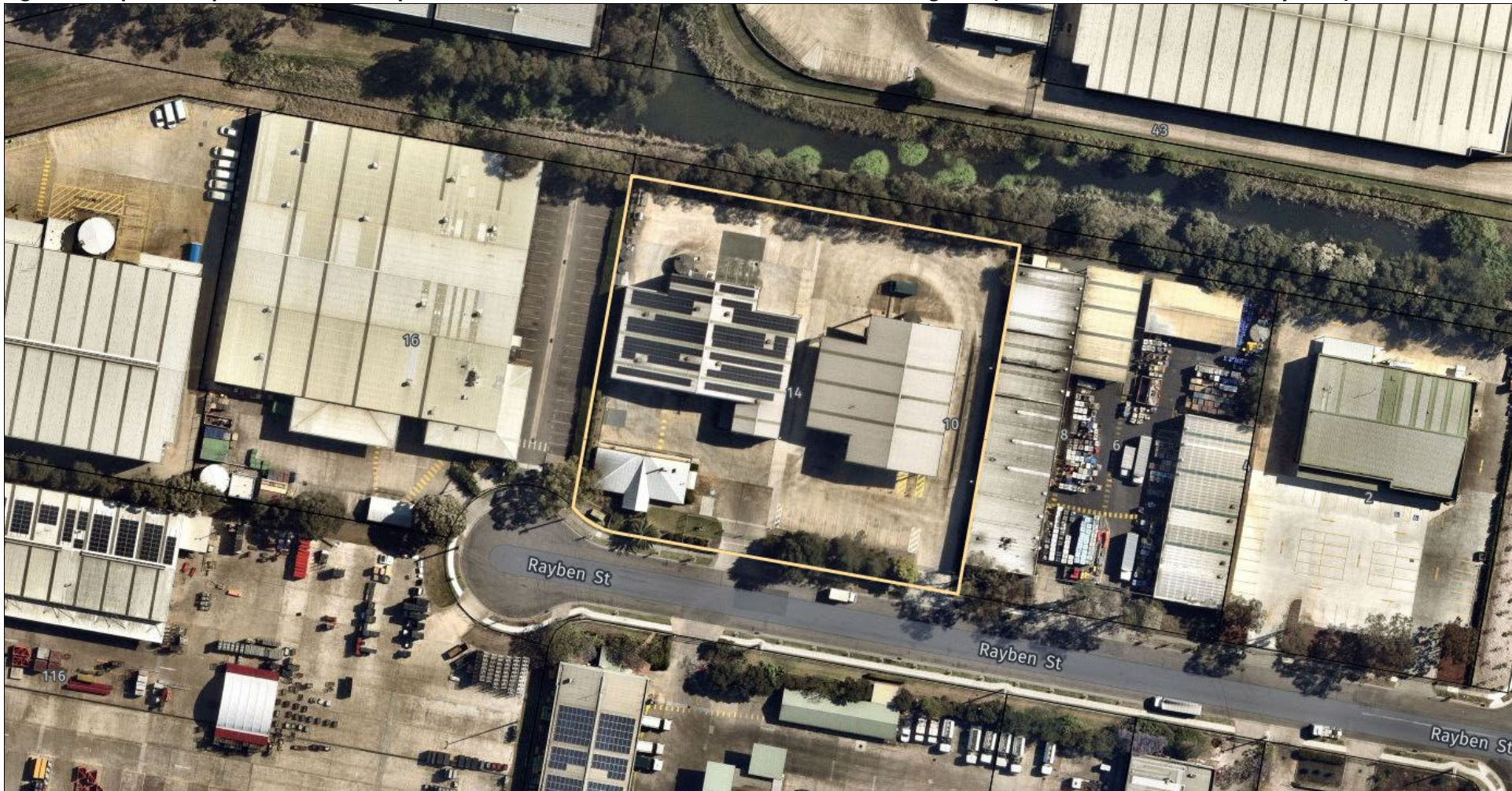
Figure 1.1. Spatial scope of the 2021 Independent Environmental Audit – JJ Richard’s Glendenning LWF (site boundaries are shown in yellow).
