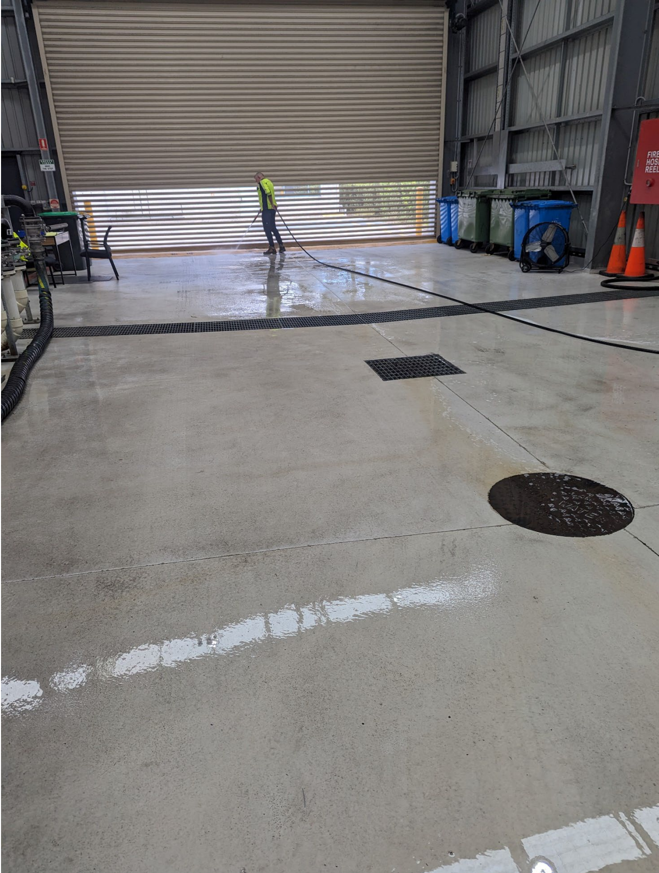
Figure D3. Grease trap and food waste unloading bay within the Organic Waste Building.
