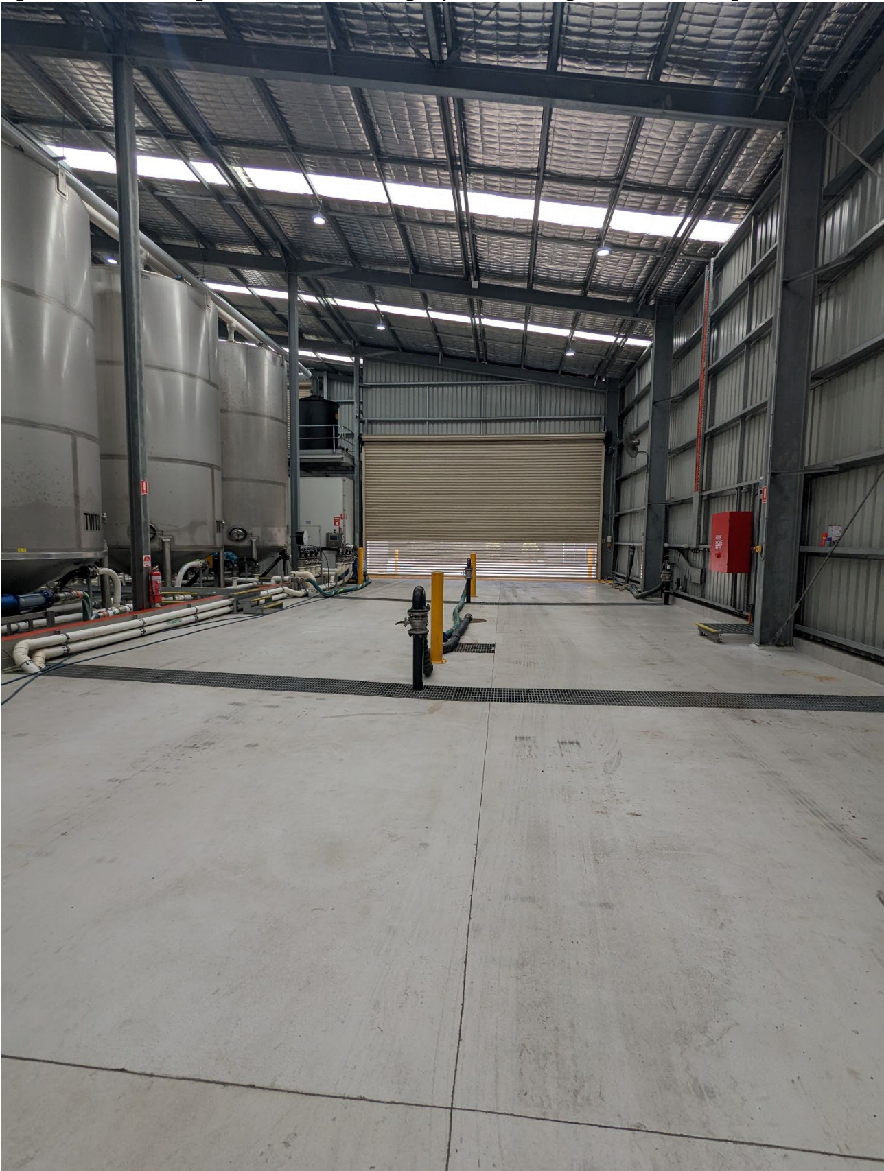
Figure D4. Treated sludge and food waste loading bay within the Organic Waste Building.
