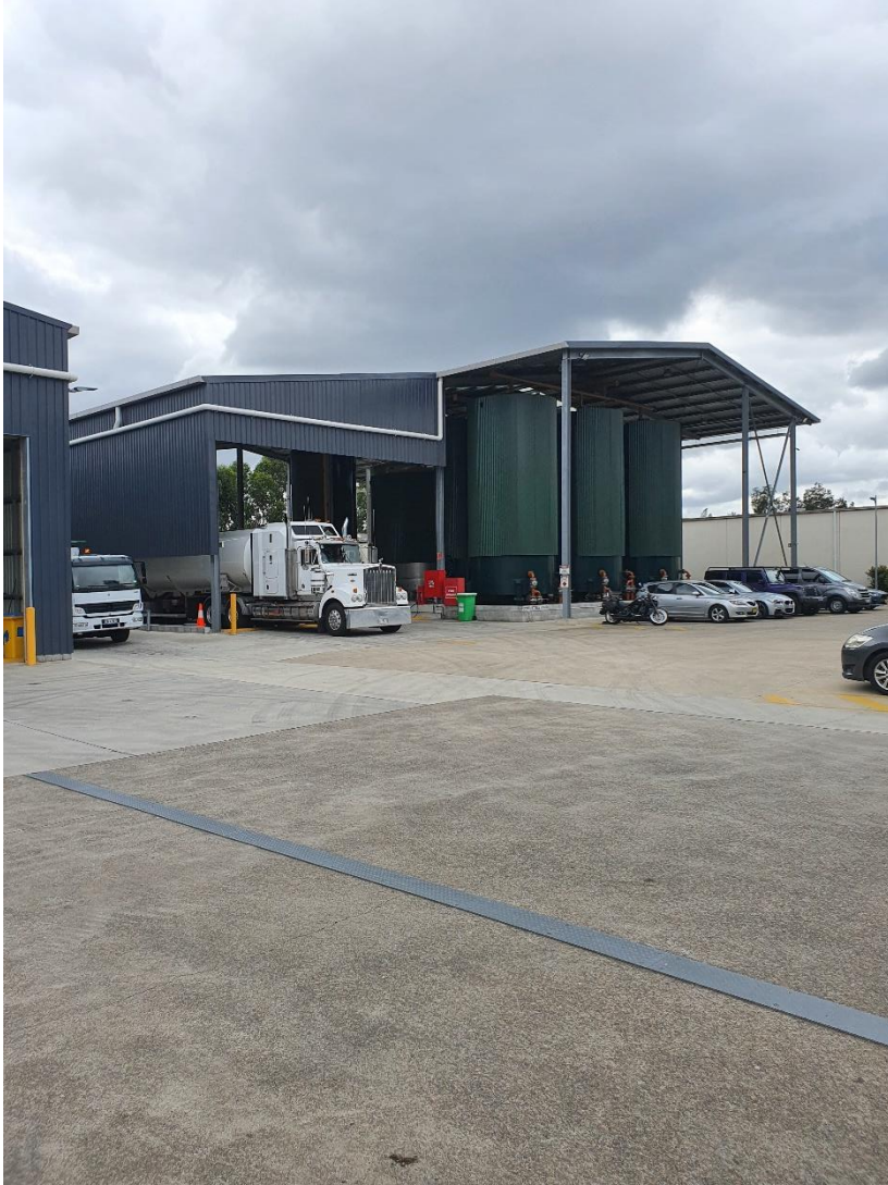
Figure 1. Front of the site showing the Used Oil Storage Roof Structure.
