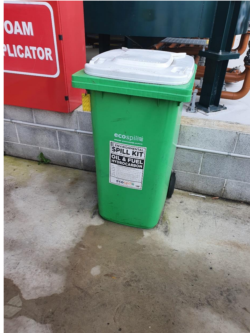
2021 Independent Environmental Audit – Glendenning Liquid Waste Facility | 77 Figure 6. Spill kits are located throughout the facility.
