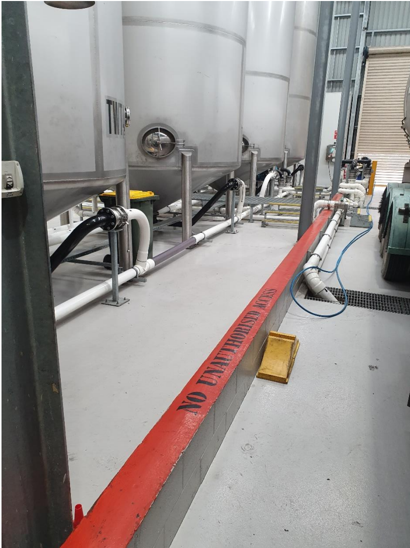
Figure 9. Bunded area of Organic Waste Building and tank farm
