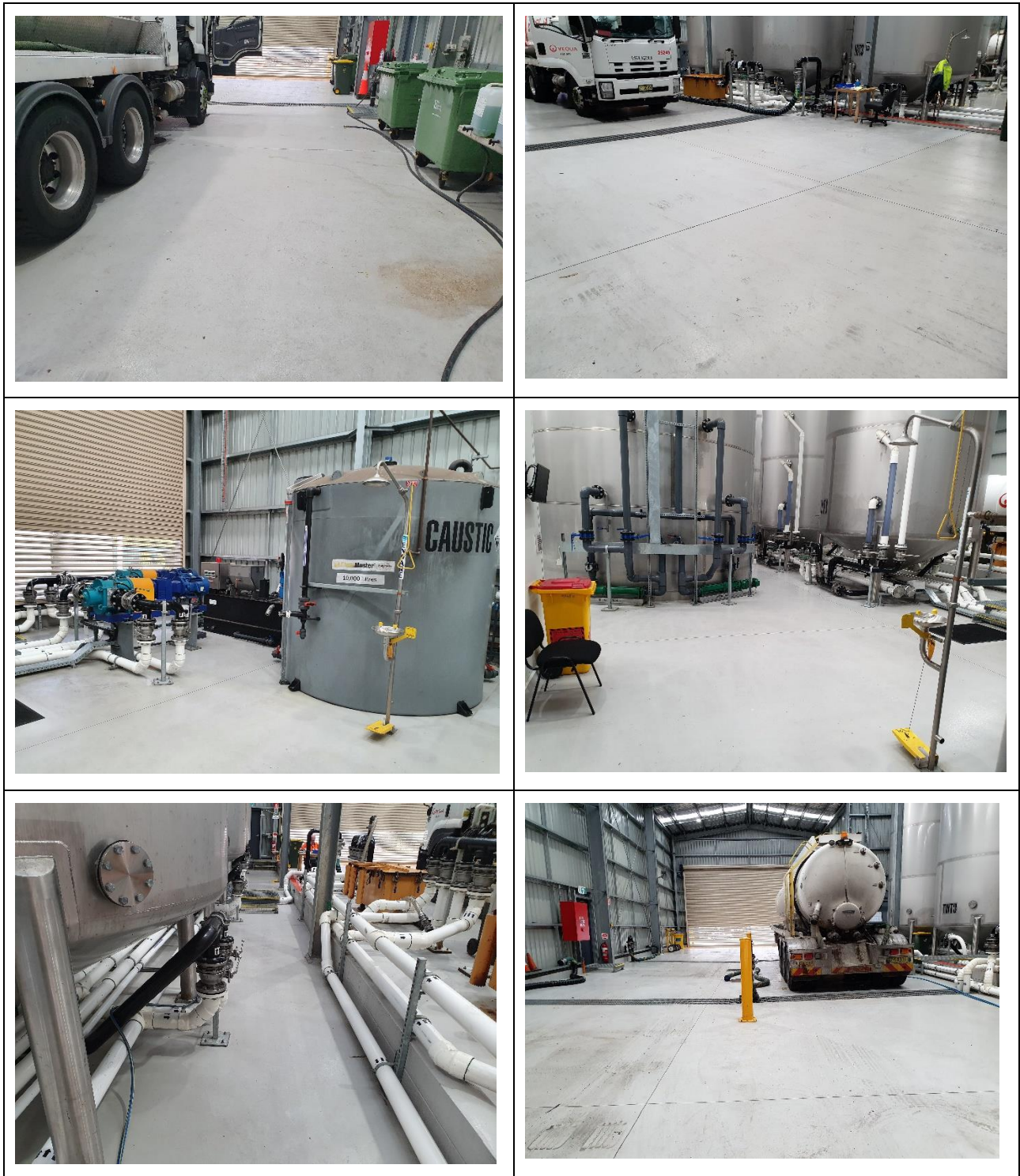
Figure 1 Organics Waste Building Surfaces
