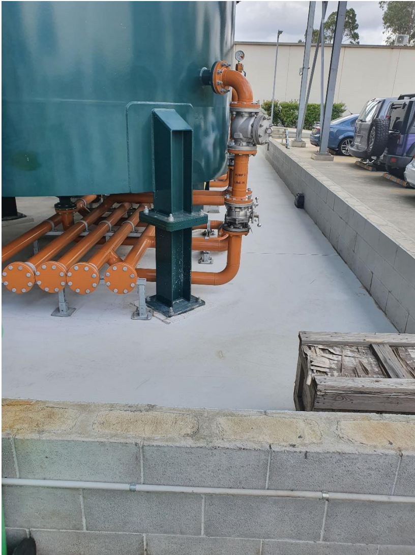
Figure 3. Bunded area of Used Oil Roof Structure and tank farm.
