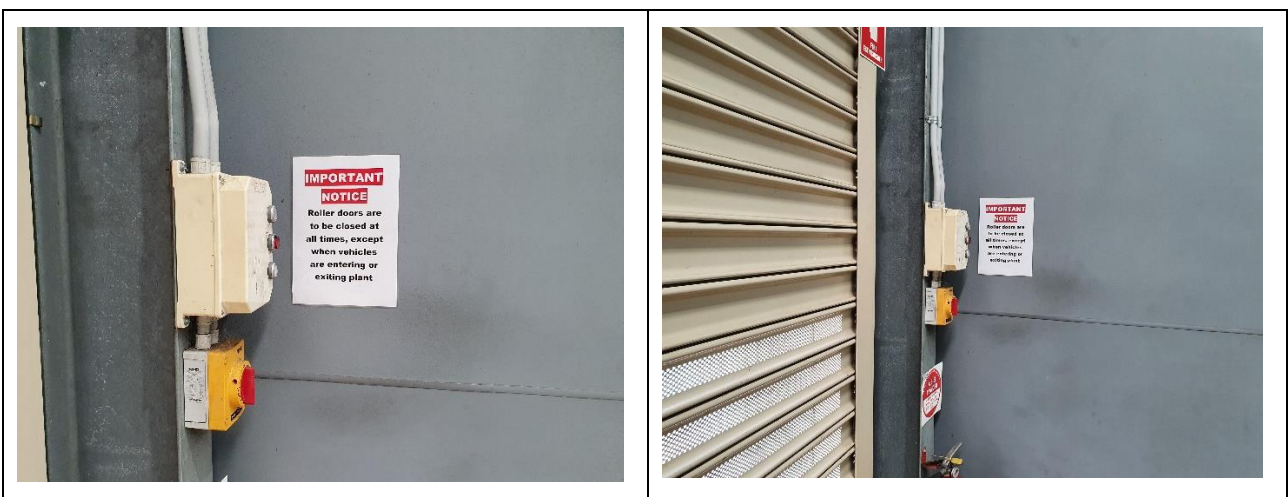
Figure 3 Organics Waste Building – Roller Door Signs
